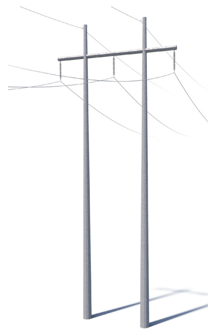
Primary 138-kV Structure
