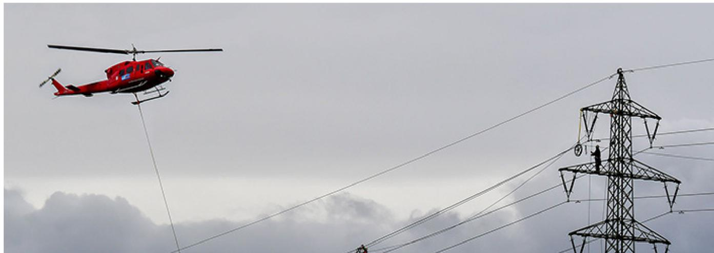
**Helicopter:** Challenging terrain or other restrictions/obstructions can make accessing certain parts of a project area difficult. In these locations, crews use helicopters to install structures, string conductors, perform line work and maintain electric facilities. Company representatives work with local media outlets to communicate these activities to the public.
