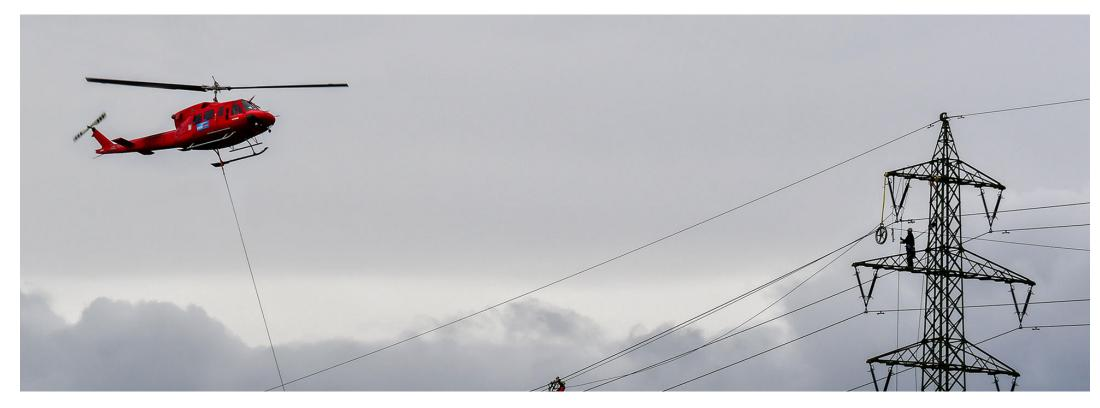
Helicopter: Challenging terrain or other restrictions/obstructions can make accessing certain parts of a project area difficult. In these locations, crews use helicopters to install structures, string conductors, per form line work and maintain electric facilities. Company representatives work with local media out lets to communicate these activities to the public.
